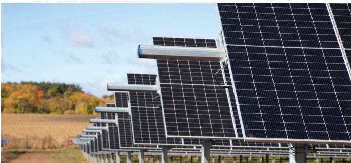
Tyto Solar under construction in Fitchburg this fall
