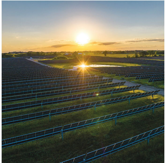
Paris Solar-Battery Park. Photo courtesy of WEC Energy Group, which is a co-owner of the project.
